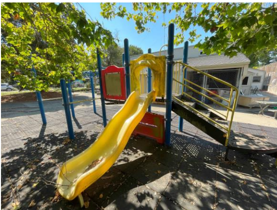
Play structure with old surfacing.
