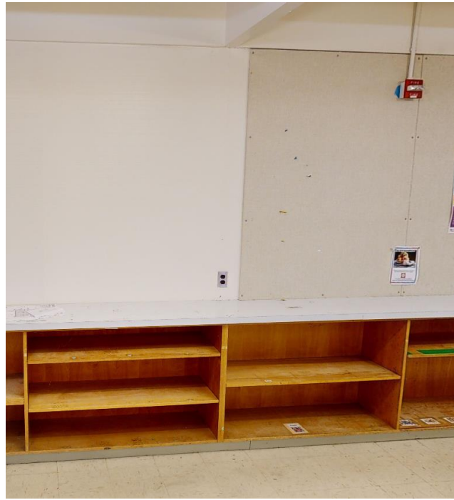
Tackable wall covering in classroom.
