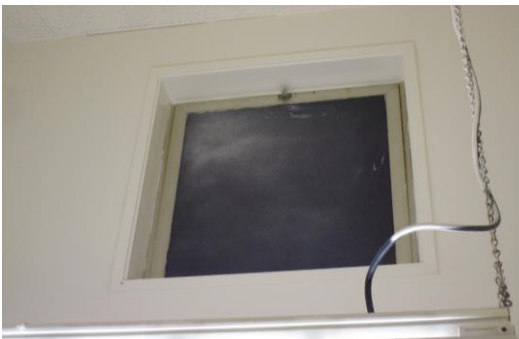
Clerestory window to attic is still in place.
