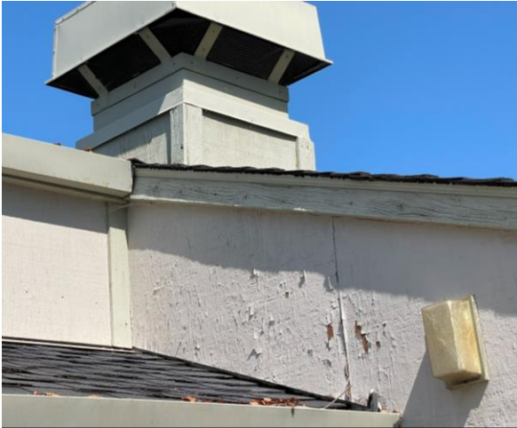
Exterior cladding is decayed. Paint is peeling.
