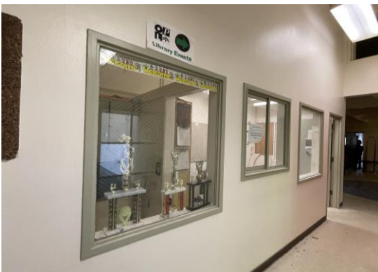
Wired glass windows in office.
