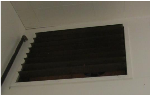
Ductwork terminates in Jalousie window.
