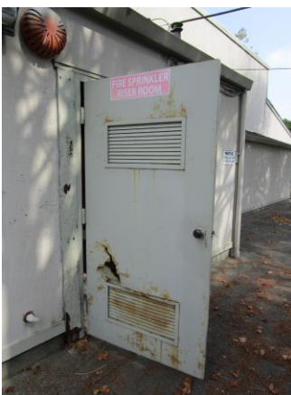
Utility closet door is rusted. Wood trim is decayed.
